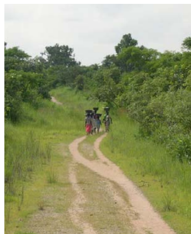
A typical road prior to rehabilitation
